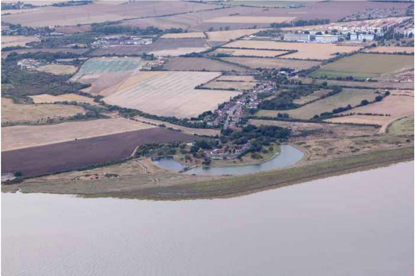
Figure 8: Aerial view of Coalhouse Fort showing its marshland setting. The East Tilbury battery is located in the small area of woodland beside East Tilbury to the rear of the Fort, whilst the Bowaters farm anti-aircraft battery is in the woodland on the left-hand edge of the photo.
