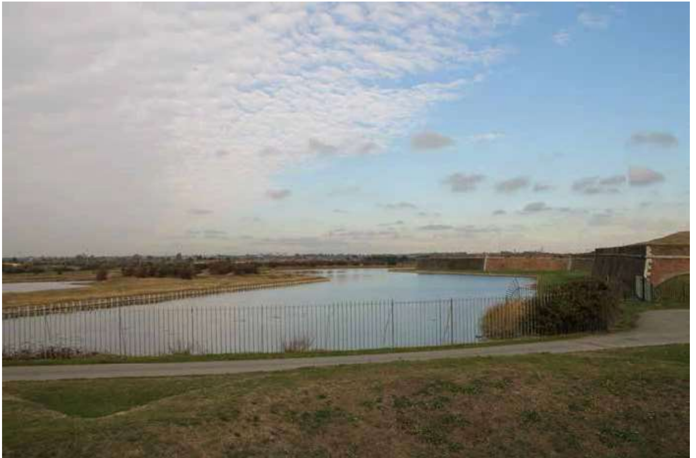
View 4: Looking north across the defensive moats to the wider marshland landscape to the rear of Tilbury Fort. The rooftops of modern Tilbury are just visible in the distance.
