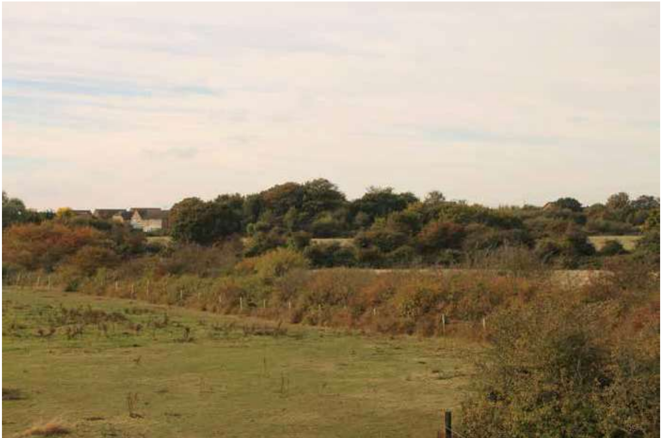
View 3: View of the battery from the east on the seawall, showing the tree and shrub growth on the scheduled monument.
