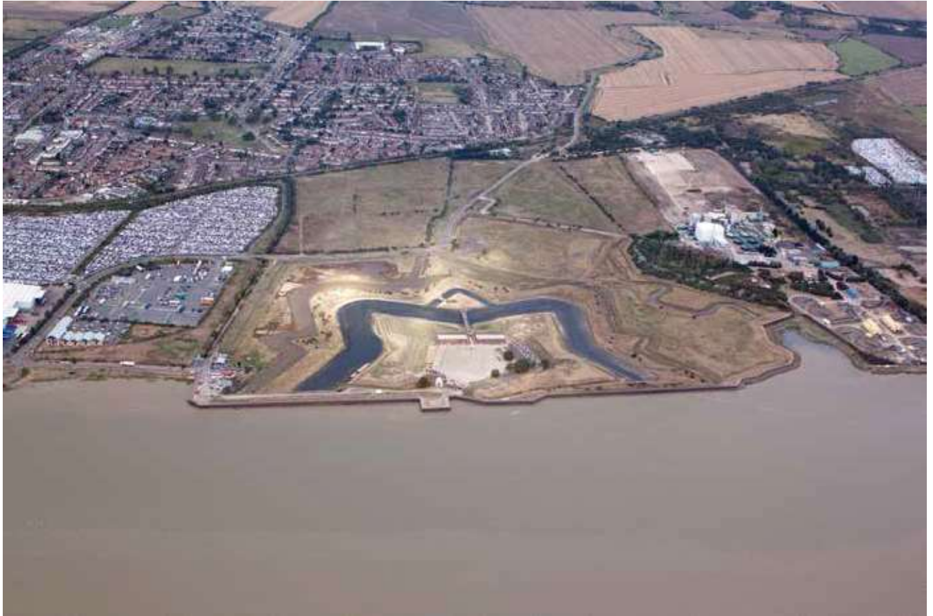
View 6: Aerial photograph of Tilbury Fort, looking northwards, showing the extent of the historic marshland, and the location of modern development in relation to the heritage asset.
